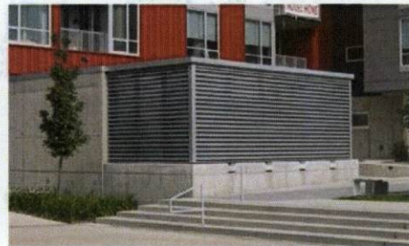
LOUVERED MECHANICAL SCREENS
